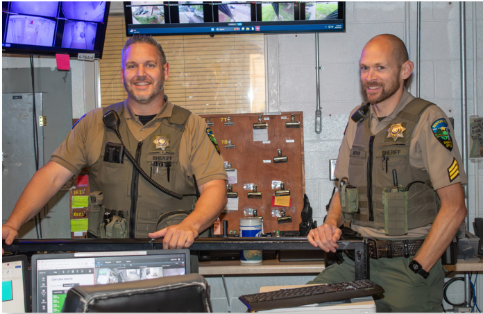
Jail Control Room
