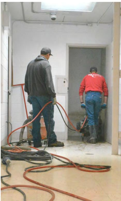
In April 2018 a water line at the Jail broke. The concrete floor had to be jack hammered up to reach the pipes. Bottled water was brought in for staff and inmates. Cost of the repairs was over \$6,800. This is just one of the many maintenance issues that must be addressed on a regular basis.
