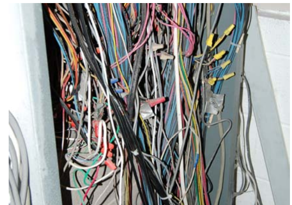
Electronics in the control room must be kept at a constant temperature.
