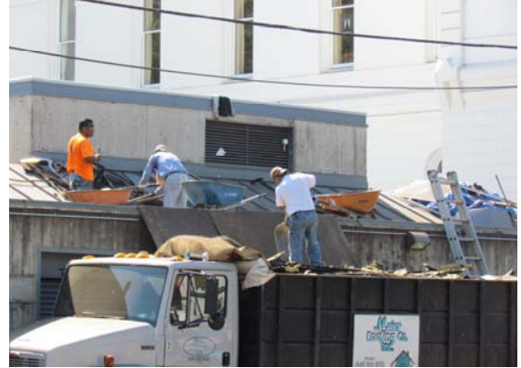
Leaky roof is repaired.
